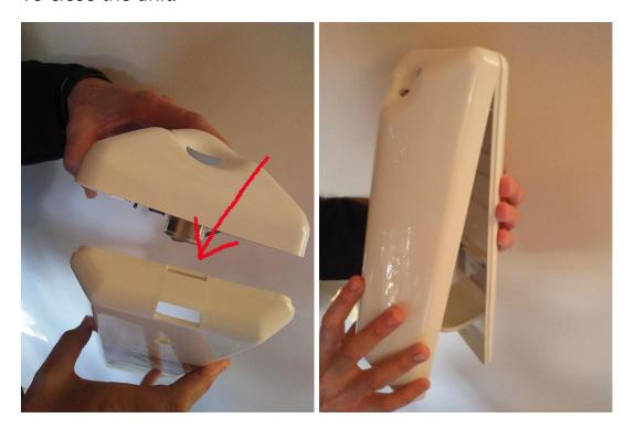
Pro Tip. When putting a unit on the wall, put the back plate on the screw first then put the face plate on. Much easier!
